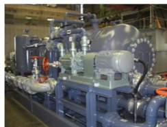
Crude oil tank cleaning
