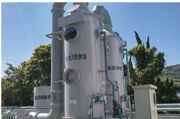
Deodorizing device by scrubber method with high deodorizing effects (Daiseki Kyushu Works)
