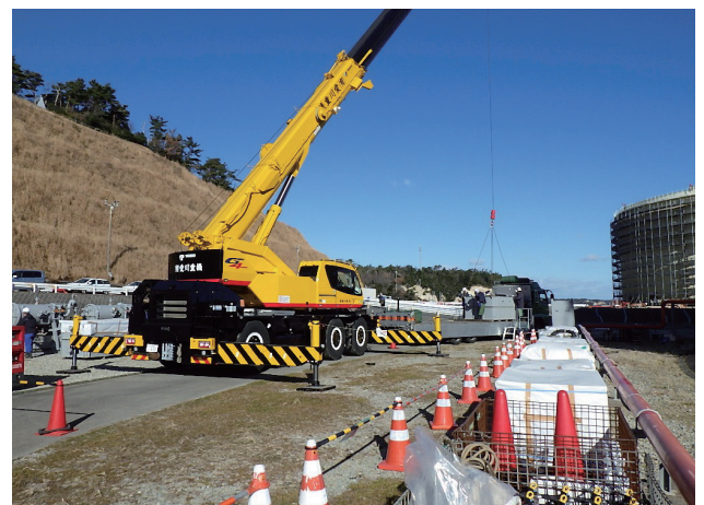
A snapshot of crane operation (System Kikou)
