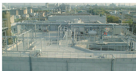
Activated sludge processing facility that can purify organic substances (Daiseki Nagoya Works)
