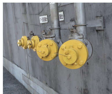
Painted pipes in plant to prevent collisions (Daiseki Chiba Works)
