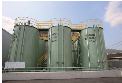
Storage tank installed with dikes to prevent wastewater seeping (Daiseki Kyushu Works)
