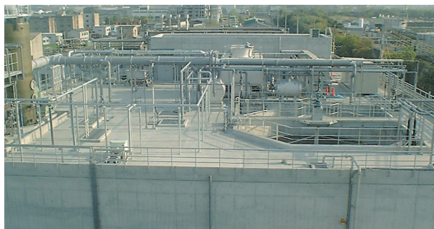
Activated sludge processing facility for biological treatment of wastewater (Daiseki Nagoya Works)
