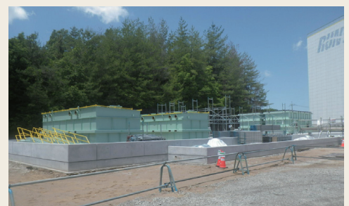
Hiroshima Works under construction
