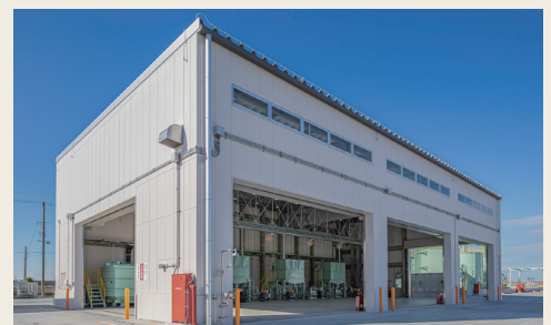
Recycled supplemental fuel plant at Harima Recycling Center
